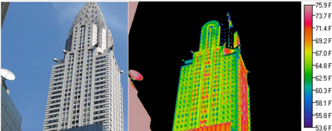
Chrysler Building (left, unaided eye and right, thermal imaging camera)
